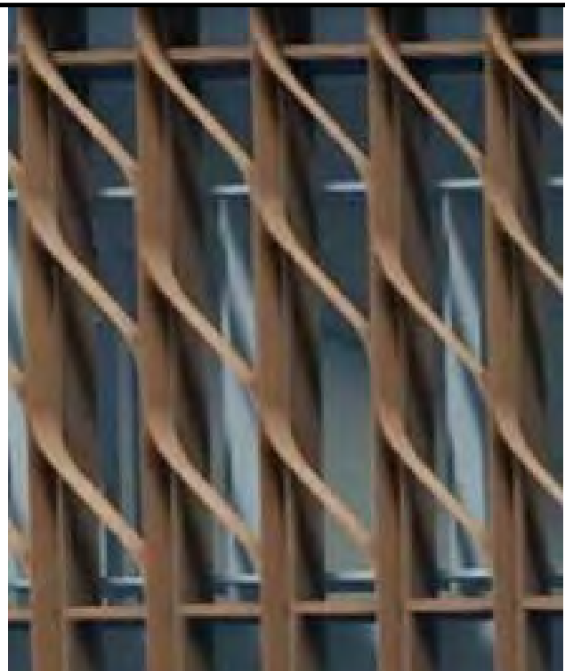
5-ALUMINIUM VERTICAL CURVED FINS SCREEN COLOUR: TO MATCH COPPER CLADDING
