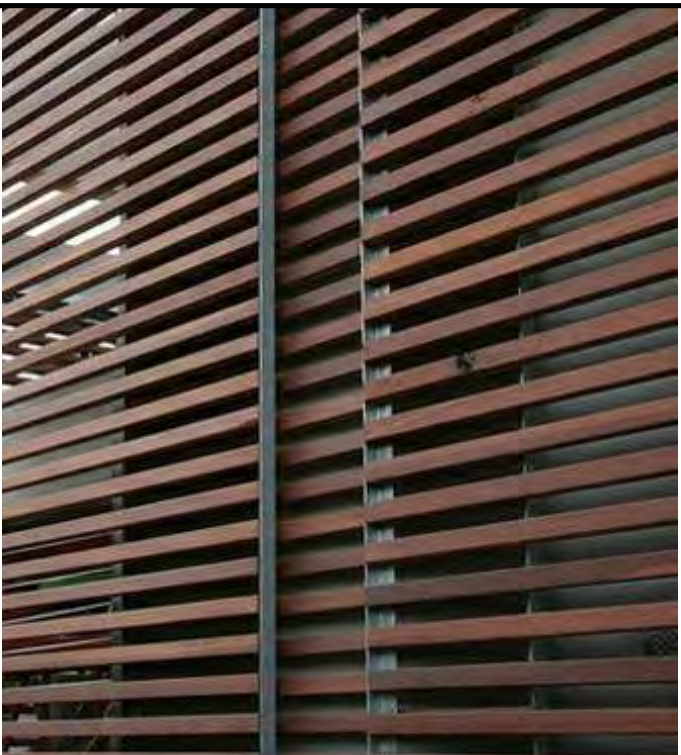
7-HORIZONTAL BATTENS SCREEN. COLOUR: TO MATCH COPPER CLADDING
